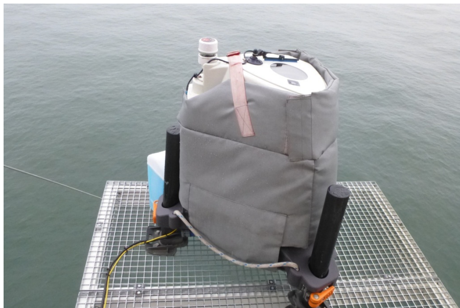
Figure 8 Installed LiDAR. North marker pointing to the right
